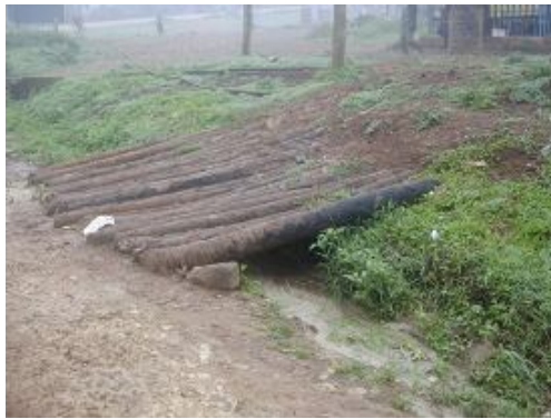
a) The trunks of Phoenix reclinata used to make culverts
